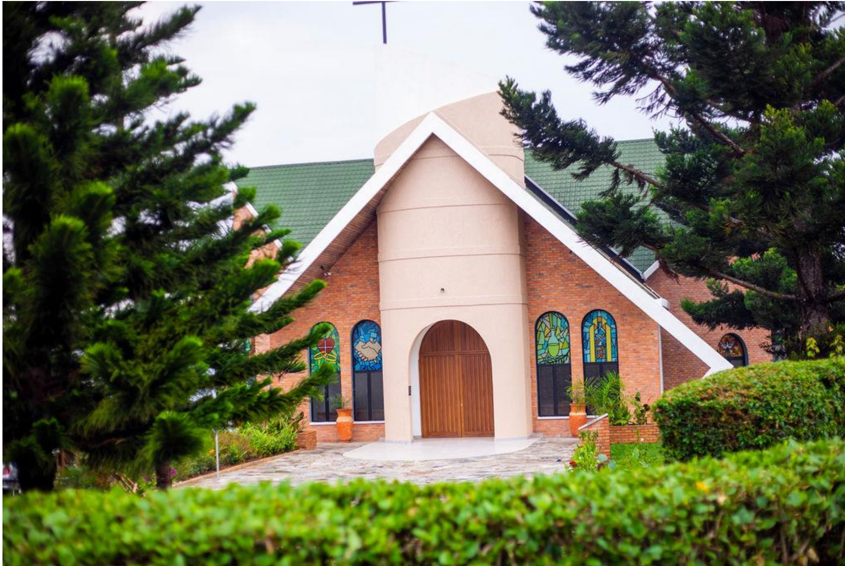
Saint Paul chapel is now refurbished and extended
